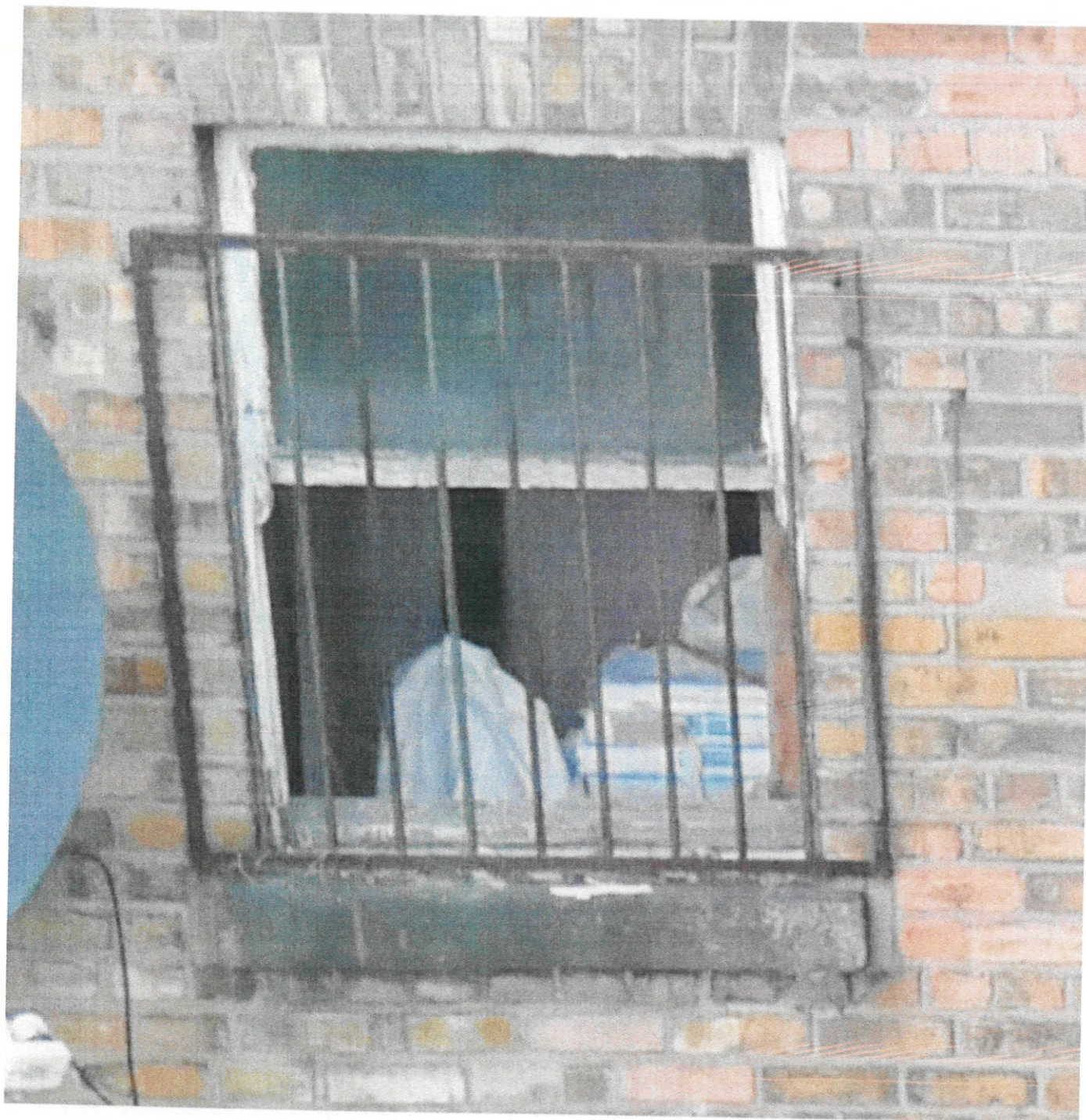
A = Bathroom window:
